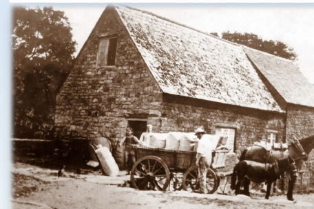
23. The Mill. The photograph shows the ancient mill in its heyday when it was operated by Mr. John Toms seen here by the wagon. The adjoining bridge was widened in 1957, but still has its sign recording that "Any person willfully injuring the bridge will be liable to be transported for life by the Court".
